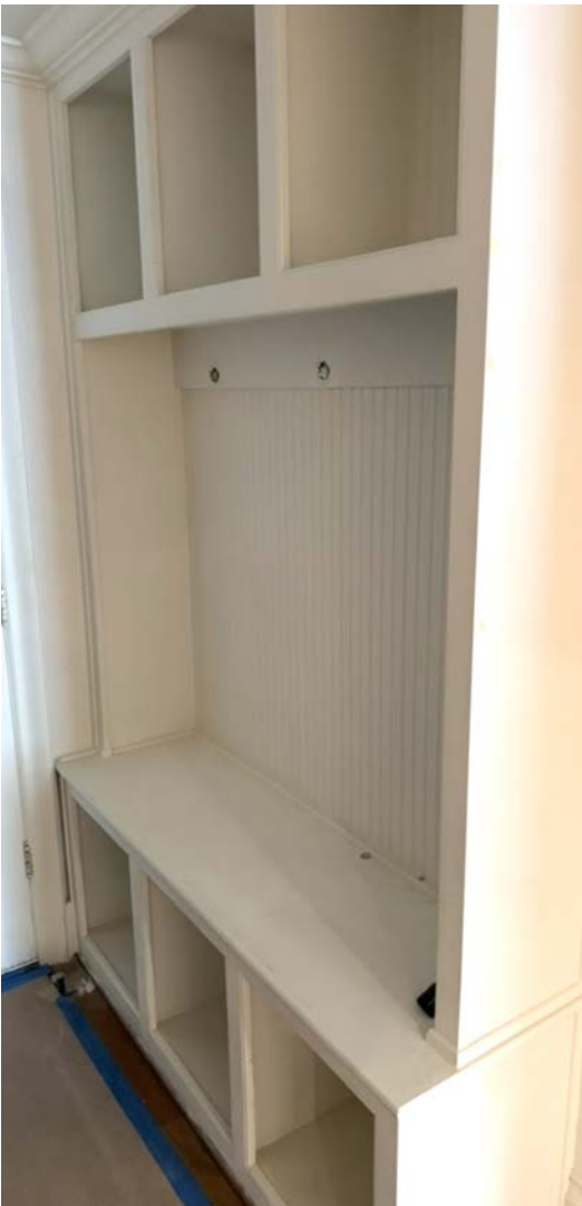
19 MUD / GARAGE ENTRY
